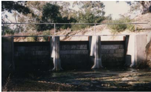
Jip Jip Weir - all boards in place 1991
