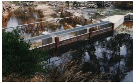
Jip Jip Weir – All boards in place with back up of water shown
